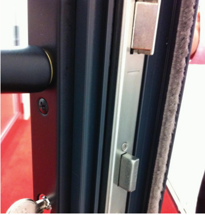
4. Latch engaged following operation 3
