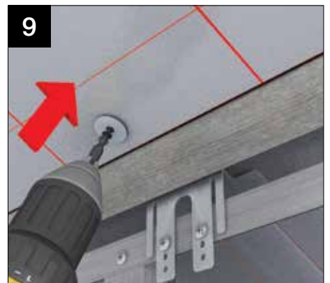
9 Fasten through the board and into the glazing bars using the drywall screw provided (3.5 x 50mm) and with a washer (kit of 25) behind the head to offer additional support to the board. Use location plan to identify board positions. Use tape LVFT045 - foil sealing tape - tape ALL joints of 25mm insulation.
