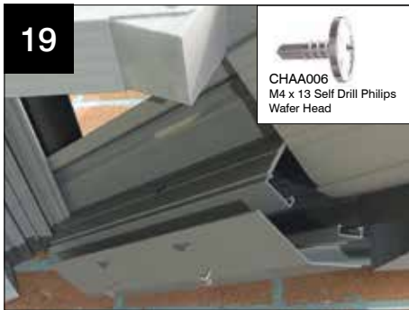
Fit valley plate at top of valley using fixings at max 250mm centres.
