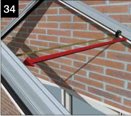
Check that the starter bar and first transom bars are parallel.
