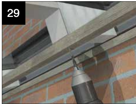
29 Fit additional battens where glazing is present along the host wall as shown.
