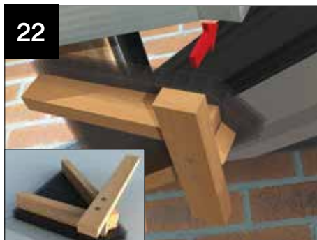
Offer up the cassette assembly into position.
