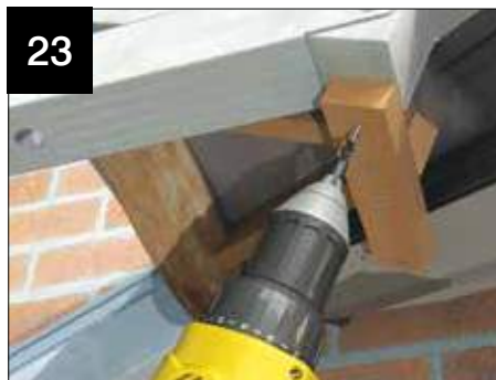
Fix into position using plasterboard screws. NOTE: when fitted, the battens should terminate at the centreline of the steel undercladding to allow for fitting of the adjacent panels
