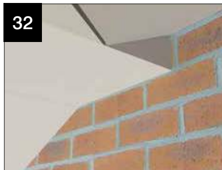
32 Now fit the plasterboard – the detail where the valley abuts the host wall should look as shown. Fitters tip: fit the small triangular segment of plasterboard shown first, allowing space for the upper adjacent board to slide in above it, as there will be nothing to screw to at this point.
