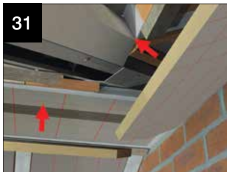
31 Fit 25mm insulation.
